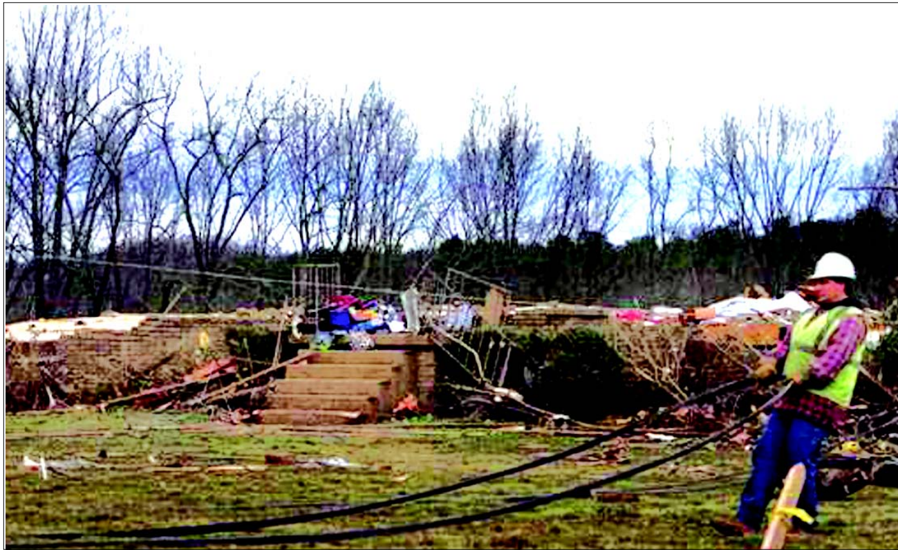
An electric worker clears away downed power lines at what remains of a home in Fairview where around 500 residents lost power in the Fairview and Pinewood areas. Coldwater, Pinewood and South Harpeth Roads were heavily affected with fallen trees and mountains of debris blocking roadways.
