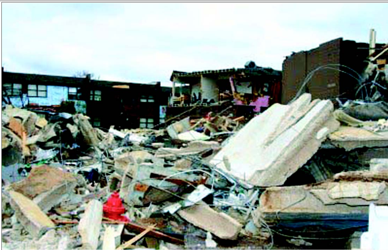
Dorms at Union University in Jackson imploded during a Feb. 5 tornado trapping more than 12 students and sending at least 50 to area hospitals. With 40 percent of the dorms destroyed, the damage estimates reached $40 million.
