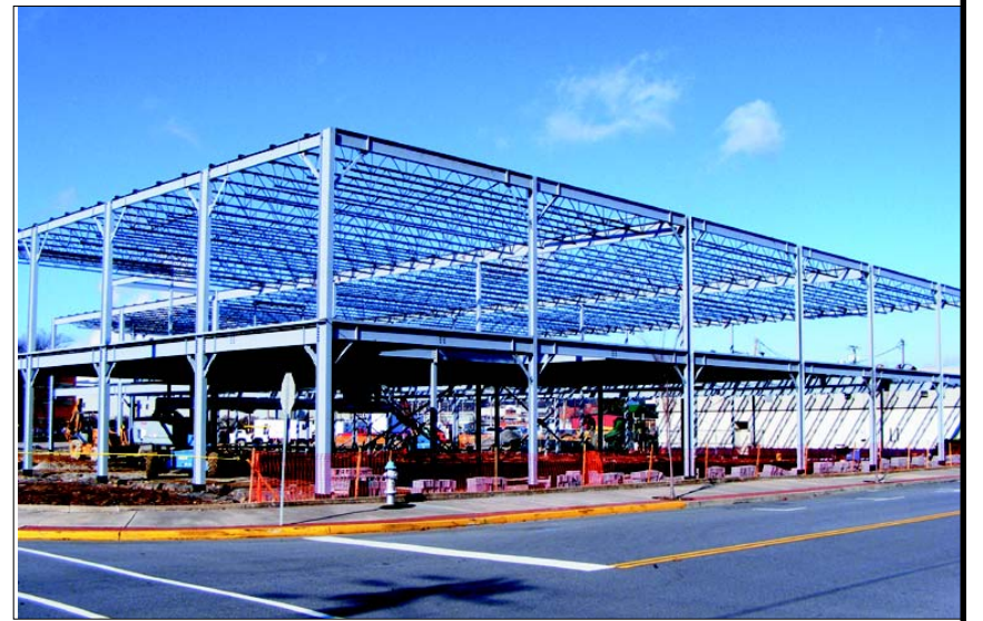
Kingsport realized $92.7 million in commercial construction and renovation. Pictured above is the Allied Health Building.
