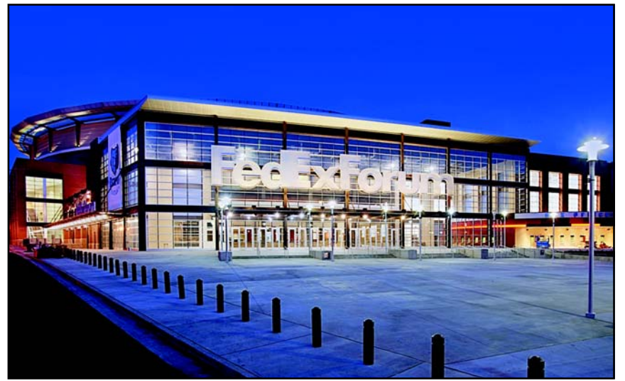
The FedEx Forum, located on historic Beale Street, is the largest public building construction project in Memphis history.
