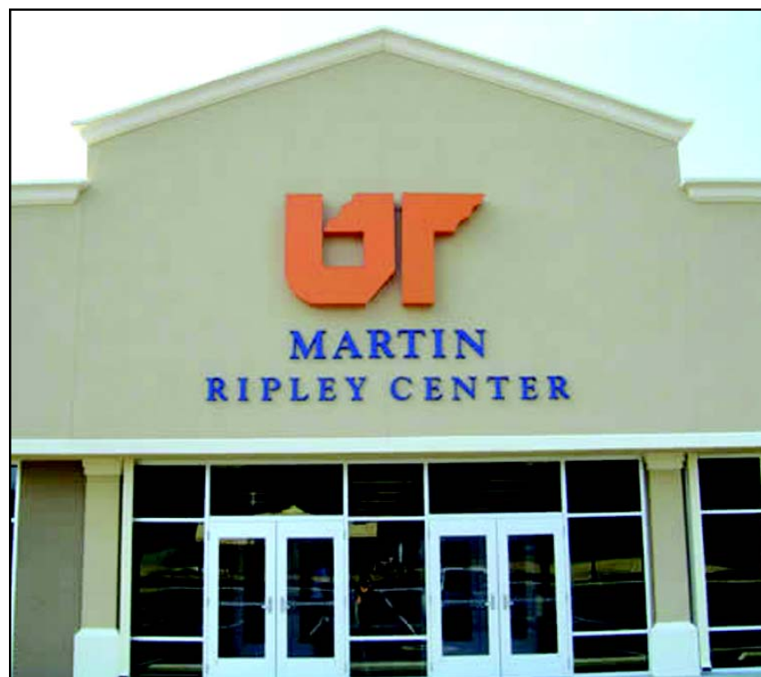
Ripley plans a complete Downtown renovation around the new UT Martin Ripley Center, a boost to their economic development.
