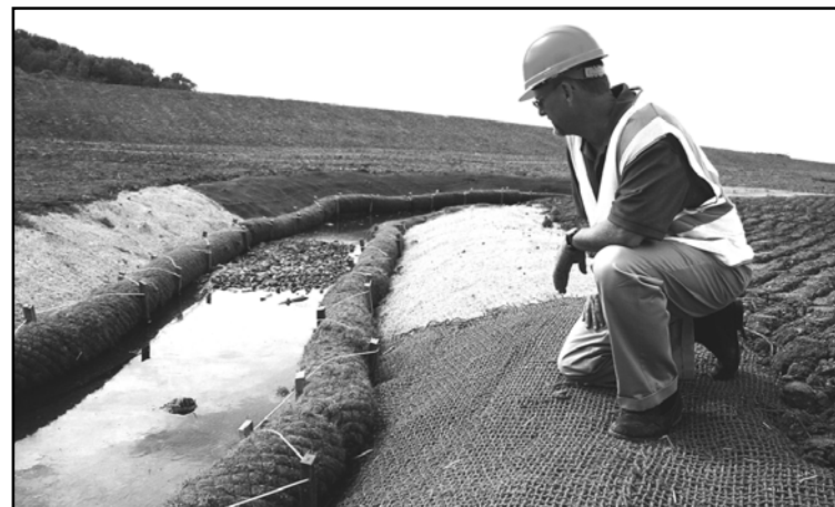
Barge Waggoner, Sumner and Cannon Inc., The Stream Relocation/Restoration for the Volkswagen Site in Chattanooga.
