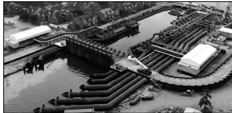
Gresham, Smith and Partners, Nashville. The New Orleans Pump Station Expansion, a project completed in Louisiana for the U.S. Army Corps of Engineers, Omaha District.
