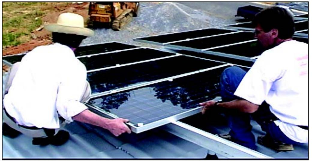
PV cells are connected in the form of flat panels that can be mounted on rooftops, canopies, or integrated into roofing shingles and other building materials.
