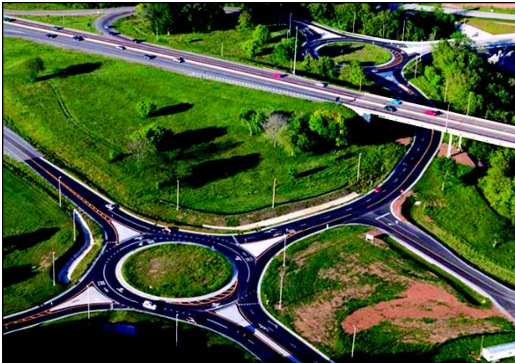
Chattanooga's Chickamauga Dam area features two modern roundabouts
