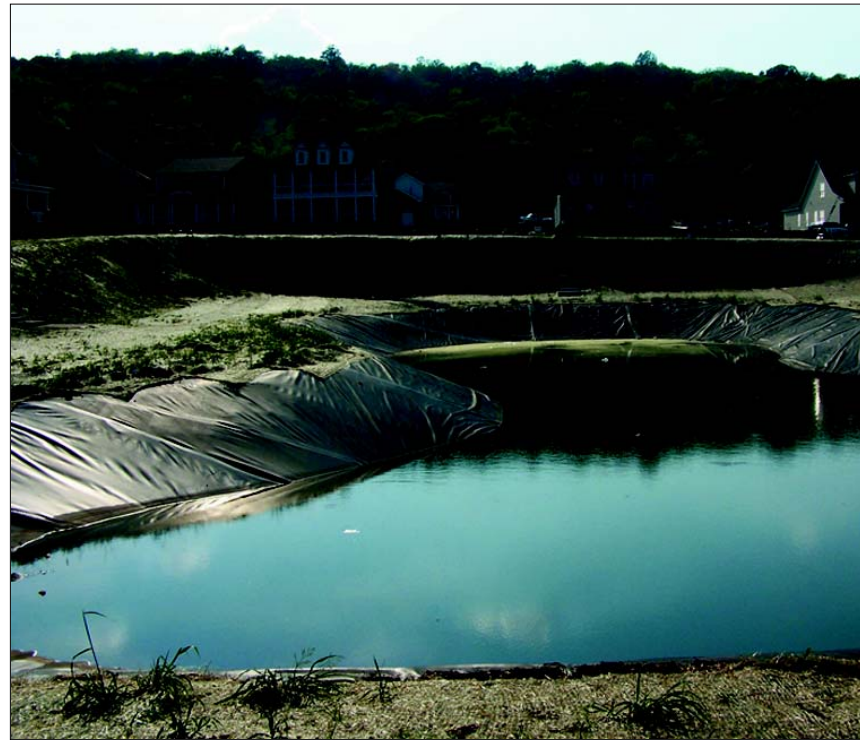
With record rainfall shortages combined with unusually high temperatures at or above 100°F, water in some community retention ponds were nearly dry during the 2007 drought.
