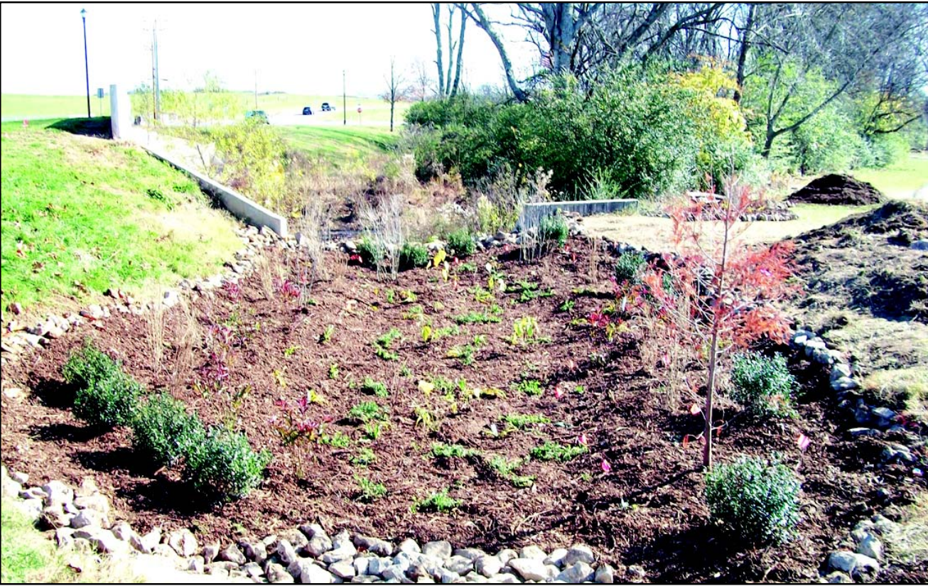
Spring Hill’s new rain garden at Harvey Park is an example of how cities are voluntarily incorporating “green infrastructure” to help filter stormwater runoff and combat environmental pollution. Stormwater pollutants can include trash and debris, sediment, paint, oil and other hazardous substances that infiltrate and contaminate lakes and streams.
