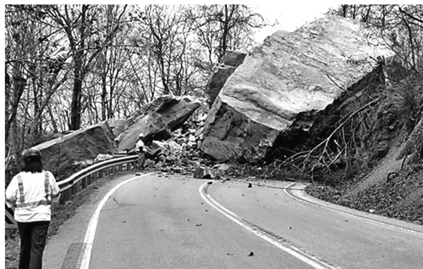
A rockslide has blocked a section of SR-108 in Grundy between Viola and Altamont and is expected to take about three weeks to clear. Detour signs will be posted along the curvy two-lane mountain road.
