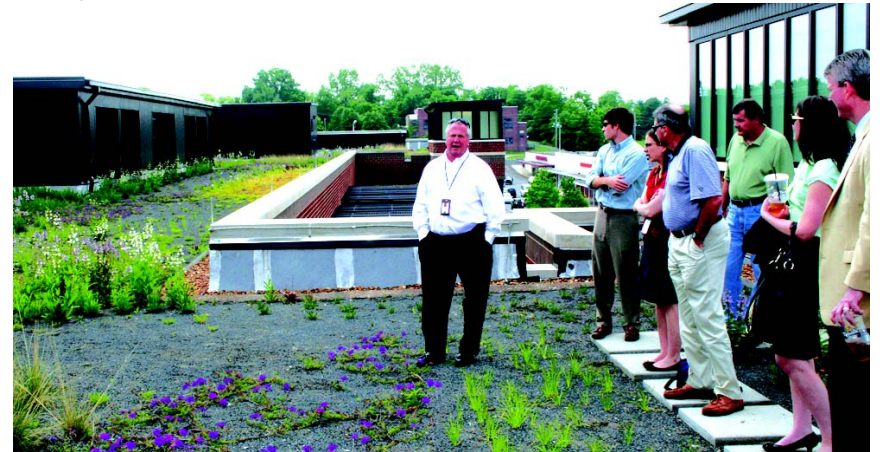
Visitors tour the green roof of the new Franklin Police Station. The roof, which includes live plant material, helps keep the 100 percent Gold Leed certified building cooler.
