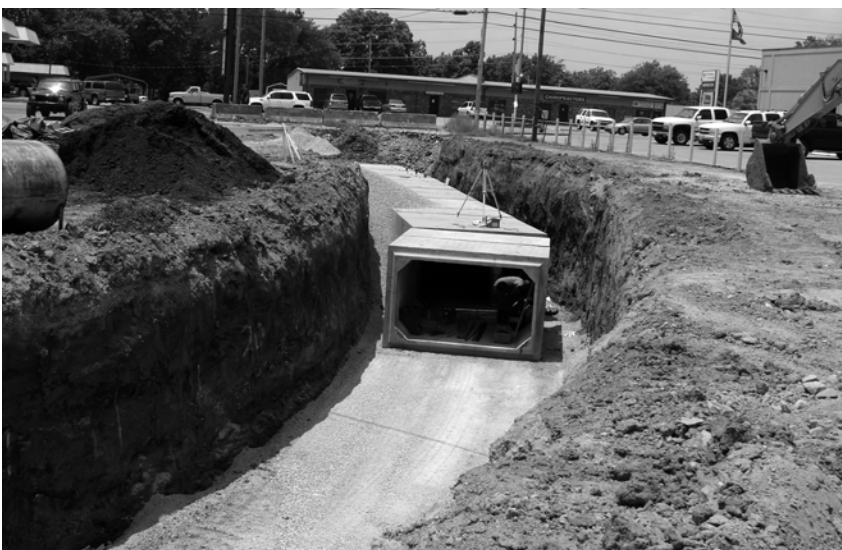
After ten years of work, Lawrenceburg is putting the final touches on the "Shoal Creek Interceptor," the 2.2 mile channel that serves as the city's main storm water drainage artery.
