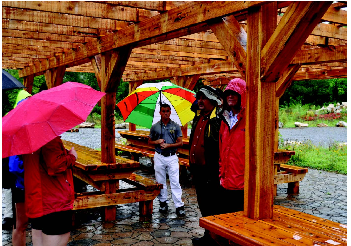
To further enhance the wetland area, Athens also added an Eastern Red Cedar Pergola.
