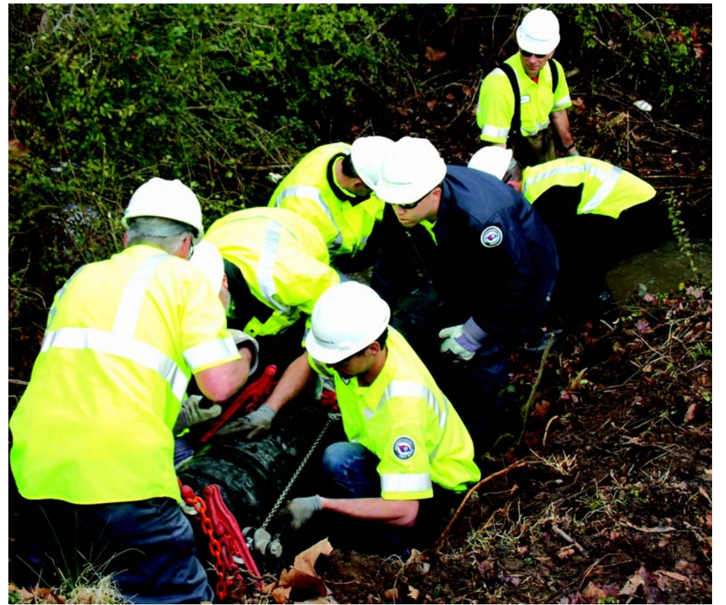
Goodlettsville's Sewer Department completed construction of an 8.5 million gallon equalization basin at the Mansker Creek Pumping Station and a sewer line rehabilitation project.
