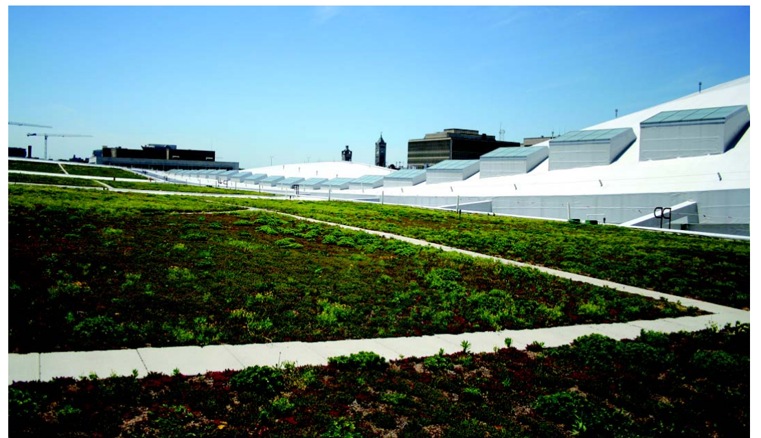
The Music City Center has a green roof spanning more than four acres. The roof sports a waterproof membrane and a 200 kilowatt solar panel grid and supports 14 varieties of vegetation along with other sustainable features.
