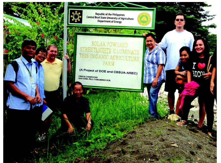
Ducktown Mayor/TREEDC President James Talley, (left) and MTAS Consultant/TREEDC Director Warren Nevad, join local students and officials in a tour of an organic agriculture farm utilizing solar-powered streetlights at Central Bicol State University in the Philippines.
