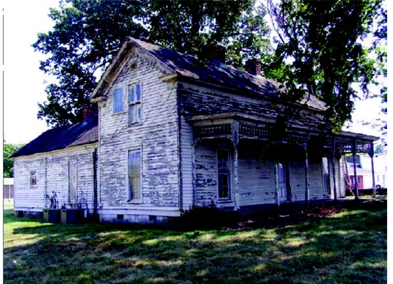
The Portland Preservation Foundation have partnered with DeRoyal Industries in Knoxville to begin restoring the Moye /Green House, which is listed on the National Register of Historic Places.
