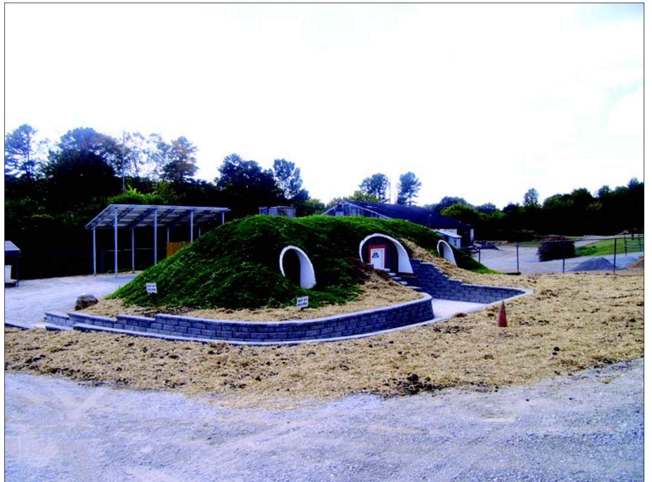
In the fall of 2013, Athens unveiled a new earthen-sheltered building—the first of its kind in the United States. Earth-sheltered means that the structure is strategically covered in 18-24 inches of dirt which moderates temperature extremes, allowing for approximately 60 percent less energy usage than a conventional house.
