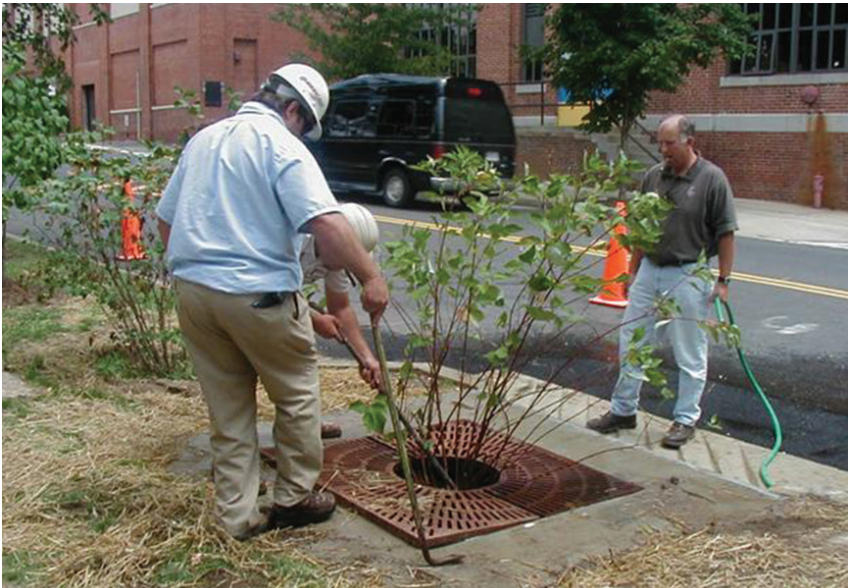
Tree well box filters will be installed in Ducktown as mini bioretention areas beneath trees. Stormwater runoff will be temporarily stored in the tree well, providing habitat for native vegetation.
