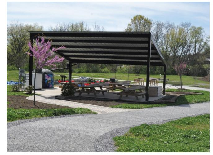
The outdoor classroom's covered pavilion area with a slanted roof channels rainwater into the cistern. The rainwater that is collected in the cistern is used to water the classroom's vegetable garden.
