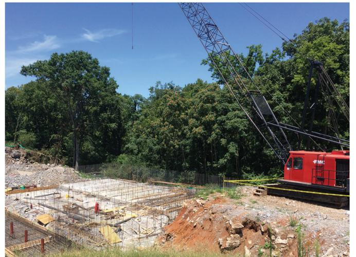
Murfreesboro officials have broken ground on construction of the Sinking Creek Plant expansion. The treatment facility expansion will increase the Sinking Creek Plant capacity from the current 16 million gallons per day to 24 million gallons per day. The expansion is expected to be completed by 2018. This expansion is critical in ensuring the city maintains its strong socioeconomic position for the population and forecasted growth in Murfreesboro 2035.
