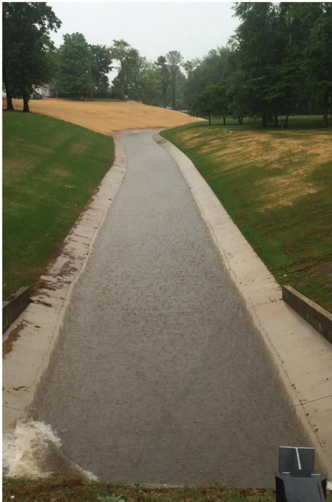
Water flows through one of the concrete collectors constructed to control the flow of water around the city. Some collectors are open air while others are tunnels that go under the surface. During the period of construction, Lawrenceburg EMA Director Joe Baxter said this collector was sometimes called "Joe's ditch." Since the mitigation project was completed, Baxter said local residents have realized how the it protects them and their property.
