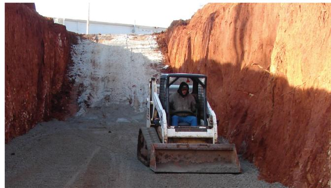
A city employee works to make room for the new culvert to reroute water from surges of Shoal Creek as part of Lawrenceburg's flood mitigation project.
