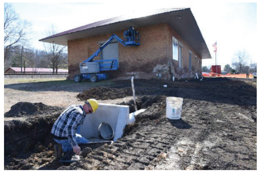
Construction crews work on the restoration of the historic Niota train depot, which also houses Niota City Hall. The depot dates back to at least 1855 and is the oldest-standing train depot in the state of Tennessee.
