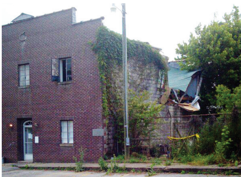
Philadelphia's old city hall was damaged beyond repair when a wind shear caused the collapse of its roof in 2013.
