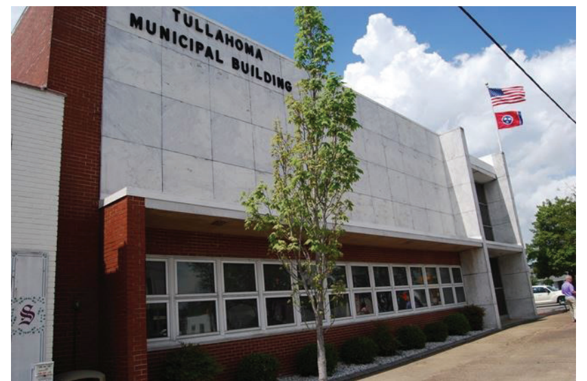
Constructed in 1951, the Tullahoma Municipal Building was recently added to the National Register of Historic Places.
