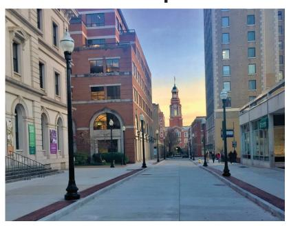
The 600 block of Market Street in Knoxville has reopened following completion of an extensive street and sidewalk improvement project that began last May. The \$493,515 upgrade involved rebuilding approximately 300 linear feet of concrete street with new sidewalks, curbs, street lights and tree wells in the 600 block. Additionally, native shade trees will be planted beginning this winter.
