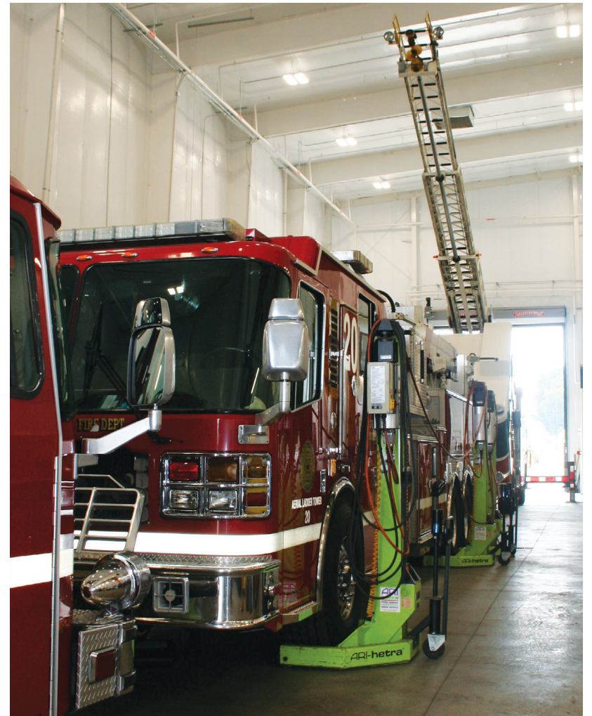
One of the new additions to the Fleet Services campus is a special bay designed specifically for the city's fire trucks. The bay is tall enough that a fire ladder can be completely extended and rotated so that Fleet Services employees can put fire trucks back on the street as soon as possible without having to work outside in inclement weather.
