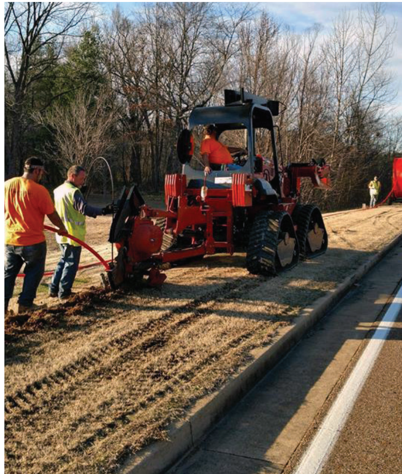
Workers install fiber optic cables in Martin as part of overall efforts to bring fiber internet access to the community. The new service will benefit local residents, businesses, and students at UT Martin.
