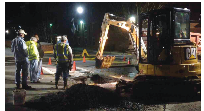
Crews in Johnson City work at night to repair a water line break.
