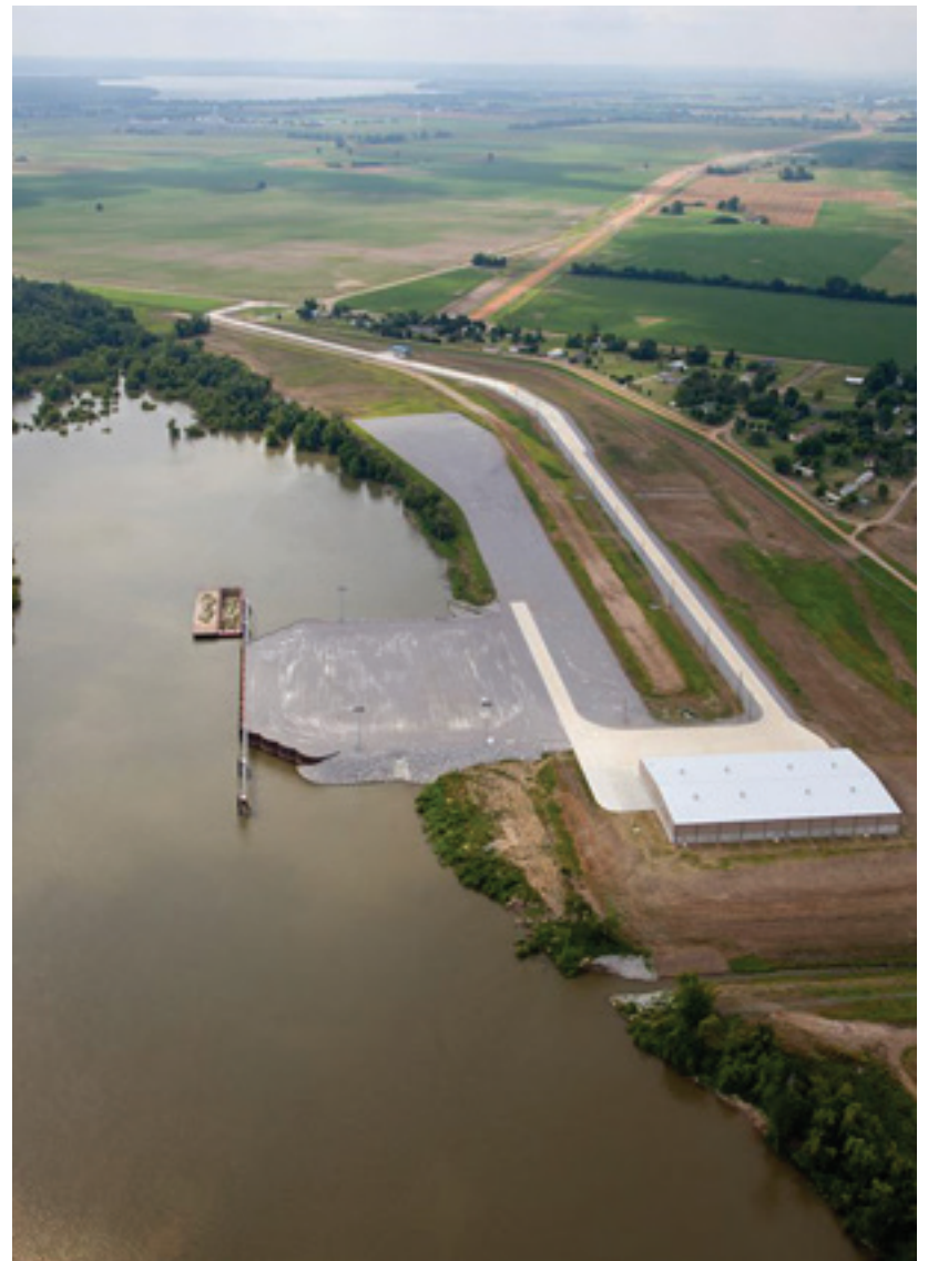
The Ports of Cate Landing, an intermodal inland port located on the Mississippi river just north of Tiptonville, is one of many important areas served by Tiptonville's water and sewer plants. Adjacent to the county industrial park, the port joins a county and federal prison as two important facilities the town services. Without a recent project funded by Community Development Block Grants, these services might have been harder for Tiptonville to deliver.
