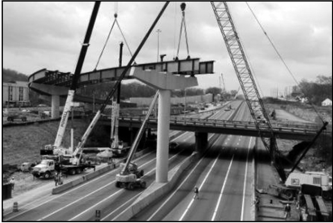
Cranes are used to lift steel bridge beams over Interstate 40 at White Bridge Road. The Nashville interchange modification project is funded through the American Recovery & Reinvestment Act.
